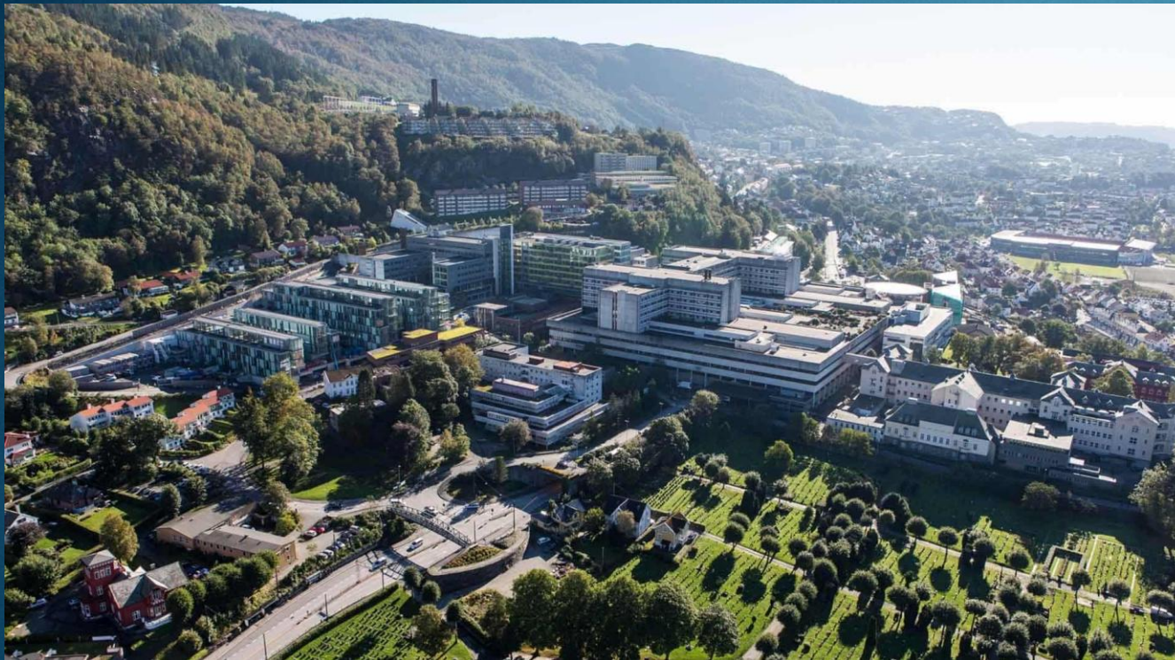
Haukeland University Hospital, Bergen, Norway
